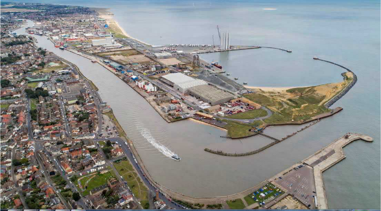
Figure 2.1: Aerial view of Port of Great Yarmouth
