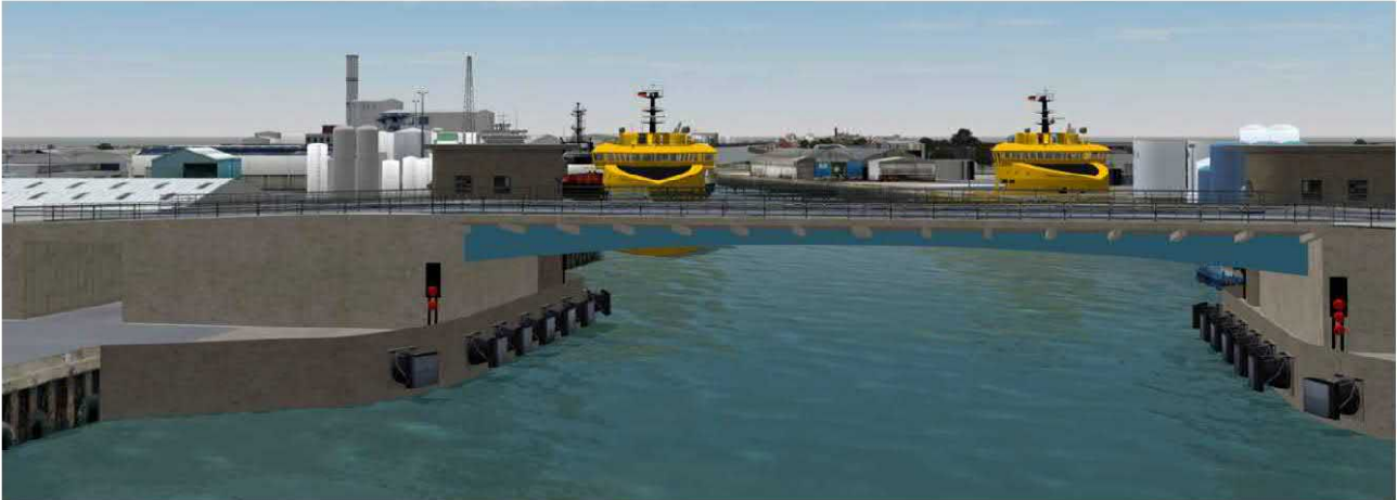
Figure 5.1: View downstream on to bridge with bascules lowered
